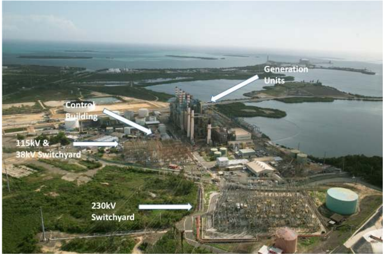
Figure 1: Aerial View of Costa Sur Steam Plant Prior to April 6 th Event (switchyard is in foreground of photograph)
