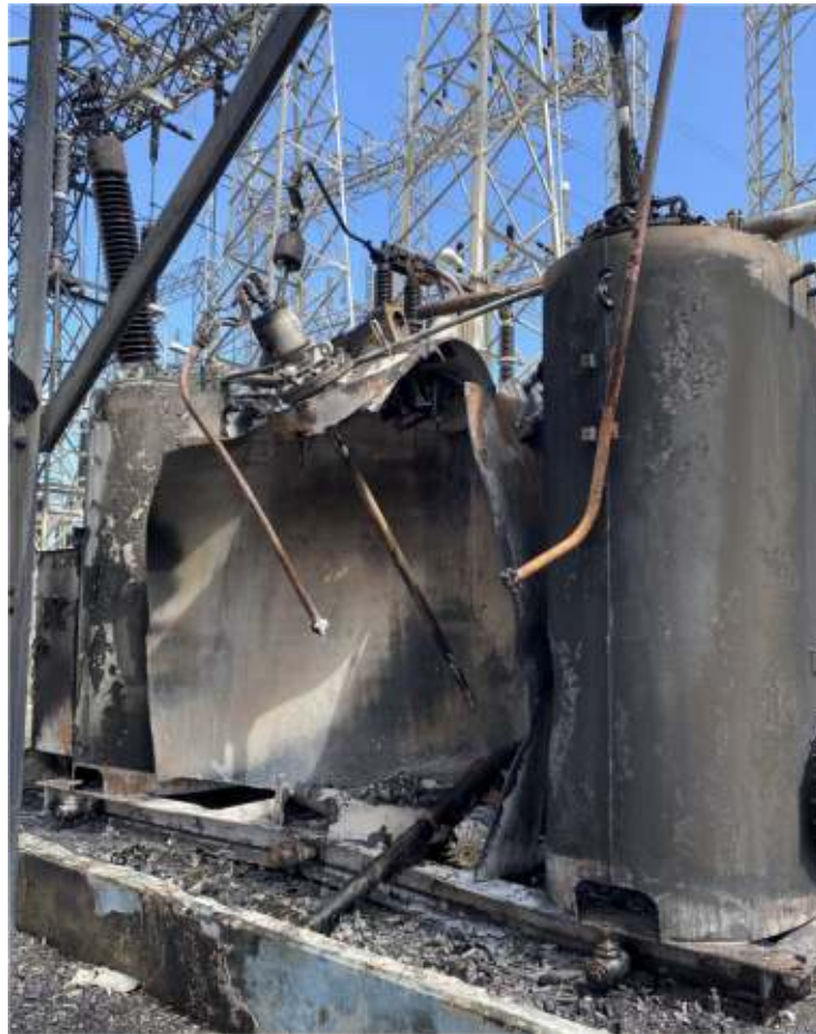
Figure 5: Damaged OCB #0082
