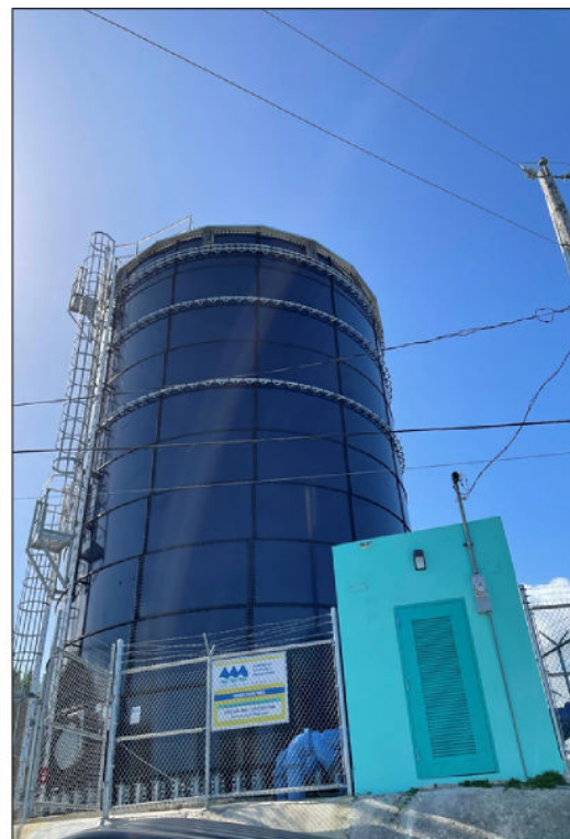
Largely repaired water tank observed in March 2022
