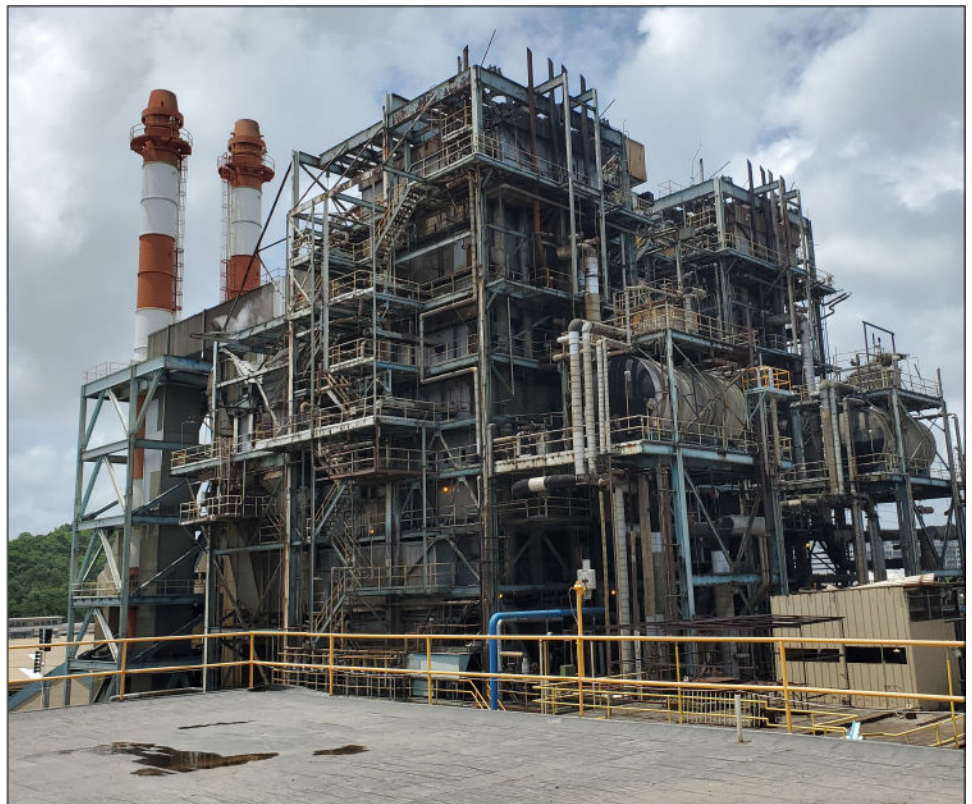
Figure 7: Puerto Rico’s Electric Power Authority Power Plant in San Juan
